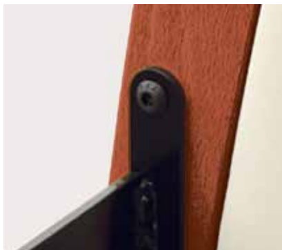
Tamper-resistant fasteners secured to metal inserts
